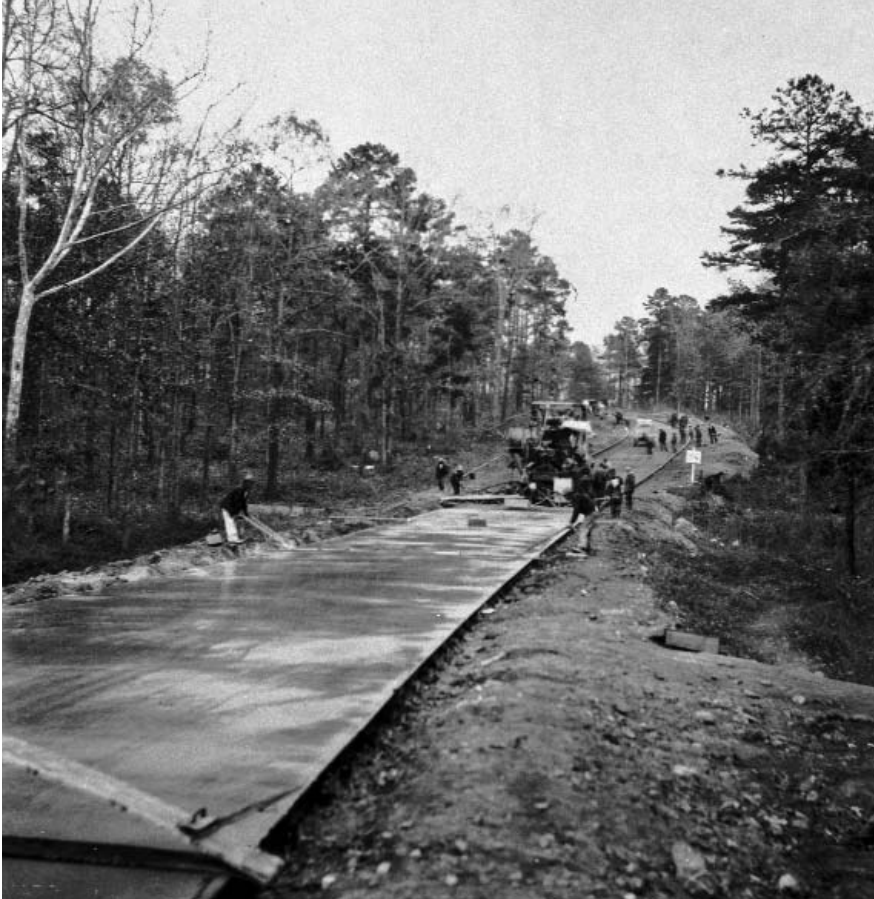
Construction of Highway 15-501 near Chapel Hill, circa 1925.
